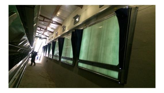
Pad room system is used in poultry houses for more efficient cooling.
