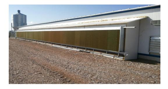
Lower case of the pad made of either PVC Plastic or galvanized sheet has also function of water reservoir. The system provided with its high capacity pump, filter and water recirculation system introduces ease of use thanks to its compact structure.
